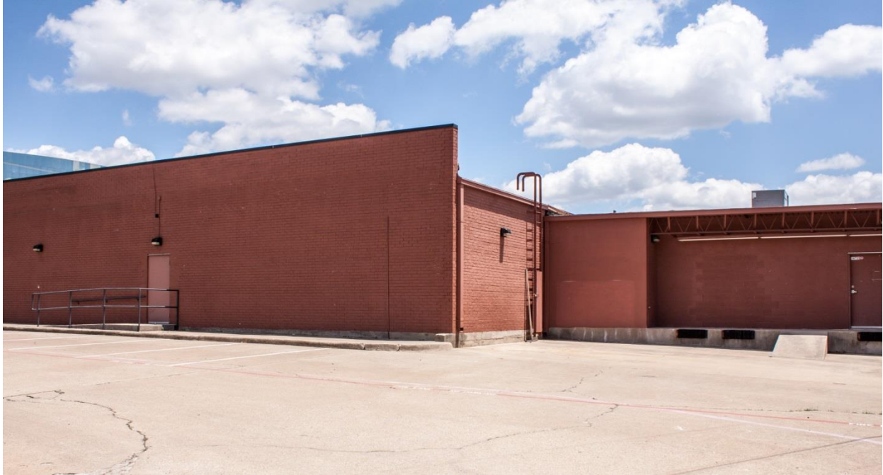
North side loading
