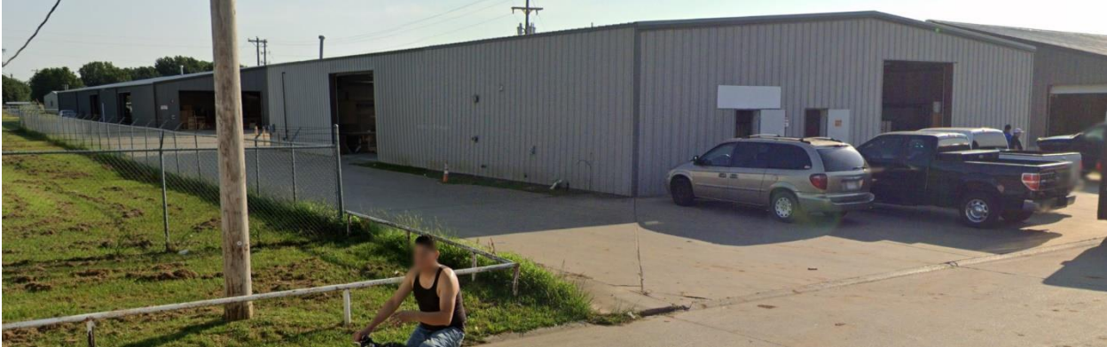
936 Prodcution Drive, front and rear buildings
